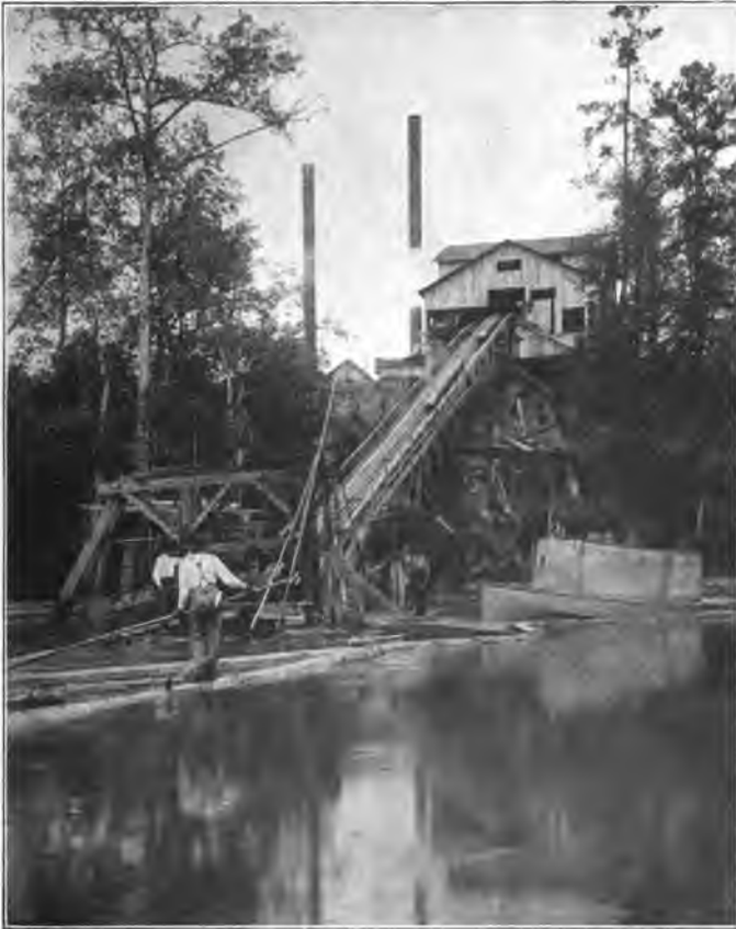
FIG. 213. LOG SLIDE AT A MILL IN SOUTHERN GEORGIA.
