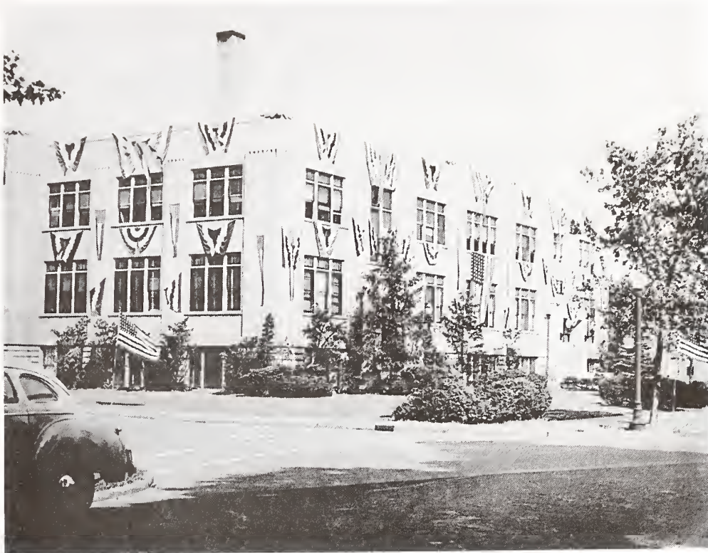
North Tonawanda City Hall, c. 1947
