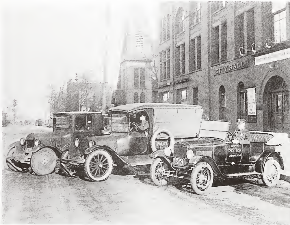
North Tonawanda City Hall, c. 1926
