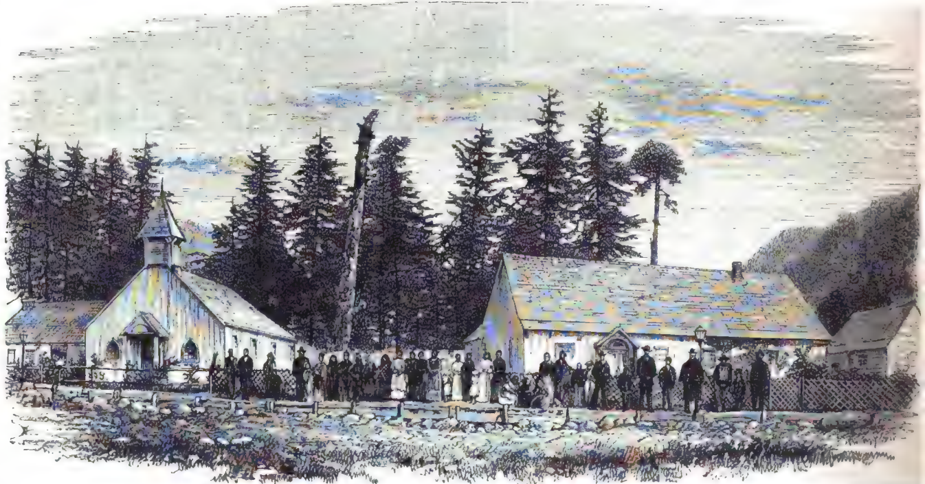
C.M.S. STATION, KINCOLITH, NASS RIVER, BRITISH COLUMBIA.
